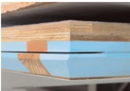
Fig. 15 Detail view of a floor structure
