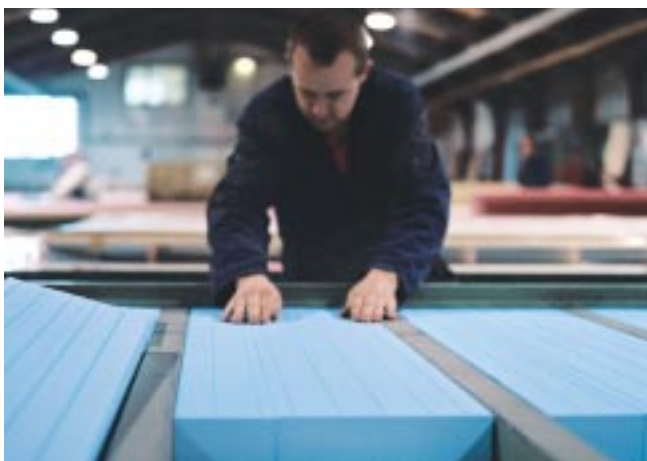
Fig. 13 Inserting the STYROFOAM boards into a floor panel.
