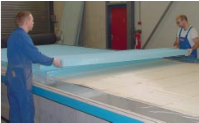
Fig. 7 Placing the STYROFOAM boards
